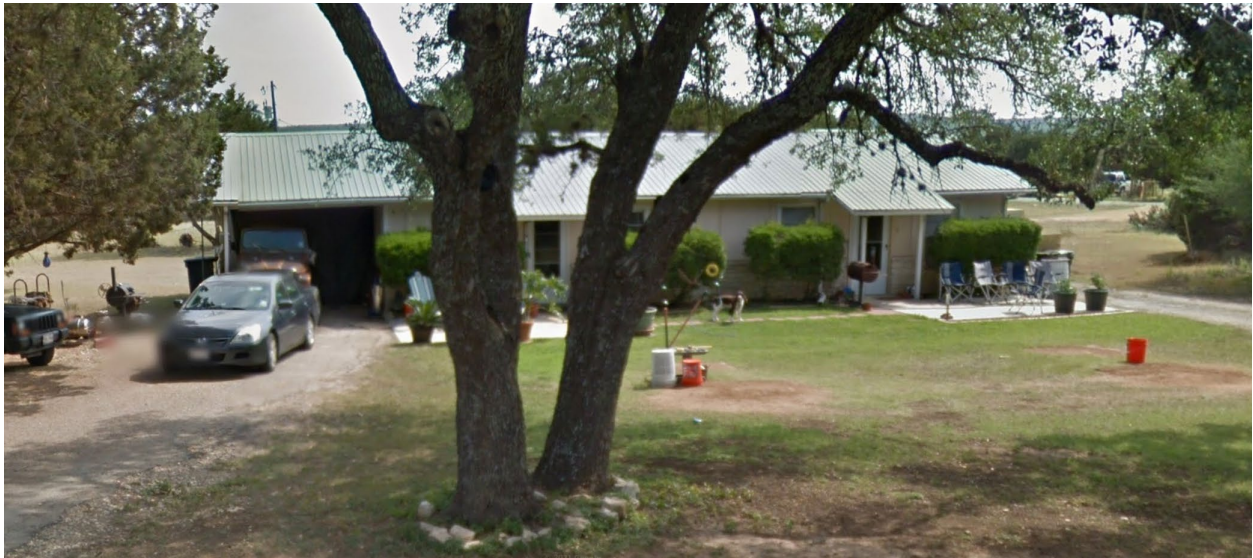
Exterior View of Existing Duplex
